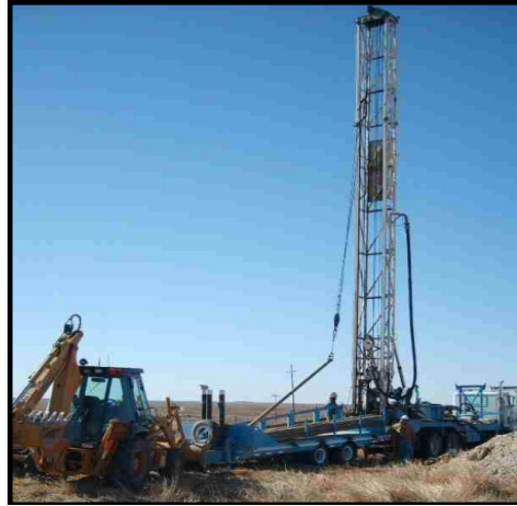
District monitor well under construction
