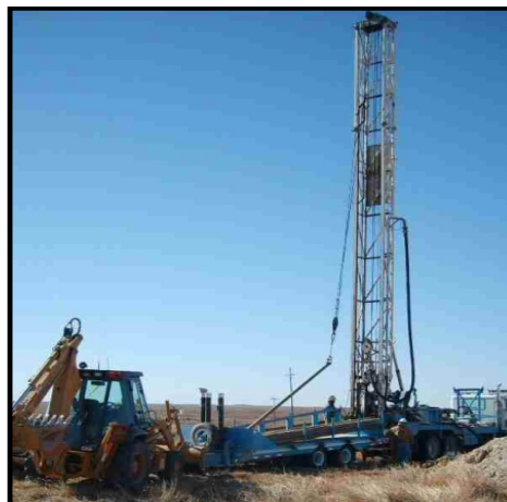
District monitor well under construction
