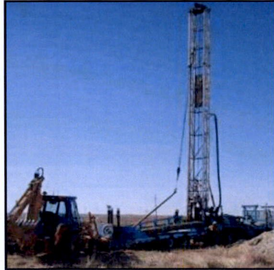
A District Monitor Well under Construction
