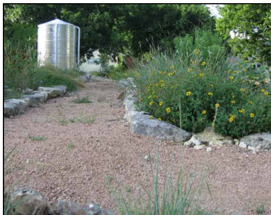
This 2,500-gallon metal rainwater harvesting tank collects rainwater from two downspouts off the Menard City Library in Menard. The water is used to irrigate the 50 plots of native plants common to that region, according to a Texas AgriLife Extension service water resources specialist. (Texas AgriLife Extension Service photo by Justin Mechell)
