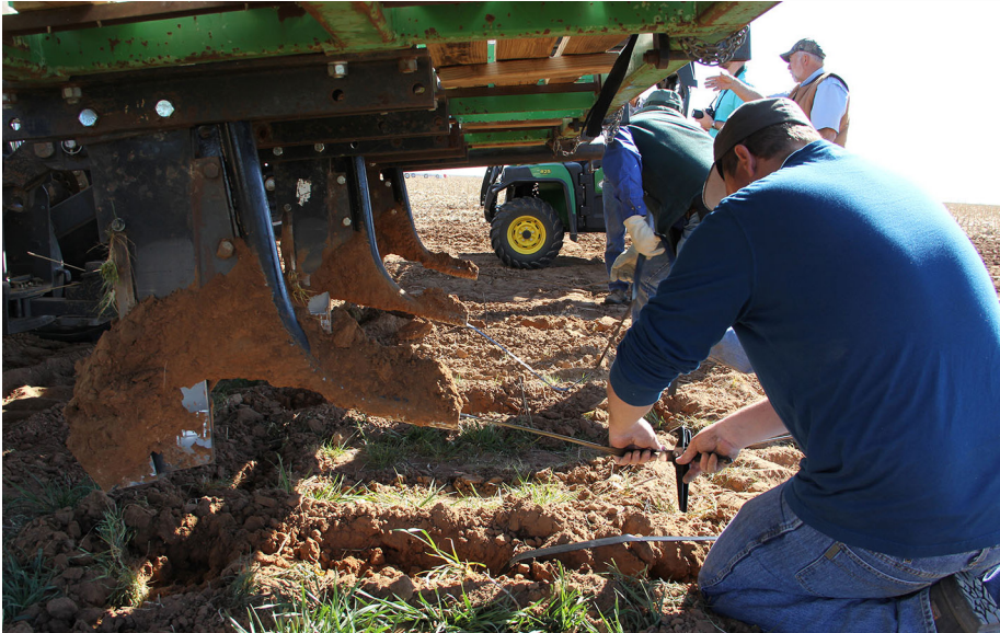
Sub-surface drip irrigation (SDI) system was plowed into the North Plains Water Conservation Center's field in February 2016. The SDI system was fully operational in May 2016.
