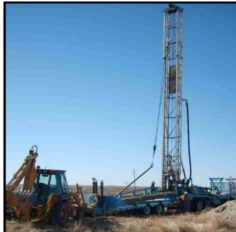
District monitor well under construction
