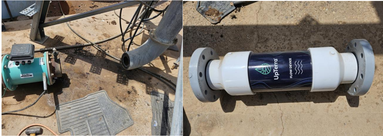
Figure 15 The UpTerra system was fitted to the supply pipe at the center of the west pivot.
