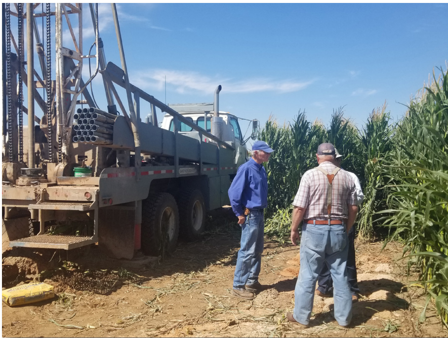
Four test holes were drilled at the WCC to find the most productive well and the most efficient location. Though additional cost was incurred to drill the test holes, the expense was minimal compared to cost of drilling a well that didn't meet the needs of the operation.
